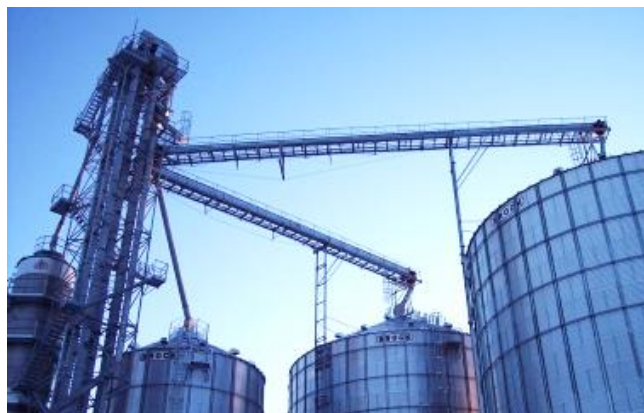
Figure 17: Chain Bucket Conveyor System
