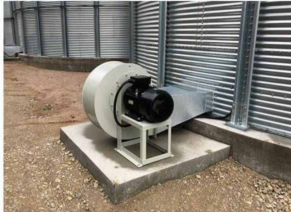
Figure 16: Installed Aeration System
