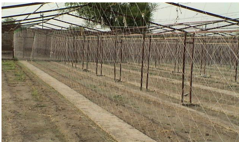
Figure 3-5: Support structure in High tunnels
